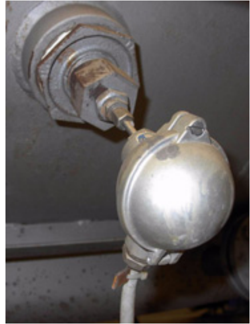
Figuur 389 Pt-100 of thermokoppeltransmitter
